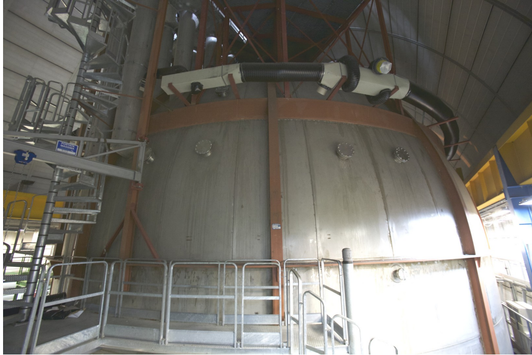
Before the thermal insulation (Mid-2015)
